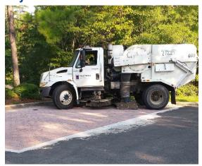
A doctoral candidate with North Carolina State University monitored the hydrologic and pollutant removal performance of PICP over a low-infiltration, clay soil from March 2014 through April 2015. Four parking stalls (540 ft2) shown at left were retrofitted with PICP to treat 1635 ft2 of contributing impervious area (3:1 run-on ratio). The PICP design followed standards outlined in the North Carolina Department of Environment and Natural Resources 2012 Best Management Practices Manual.
