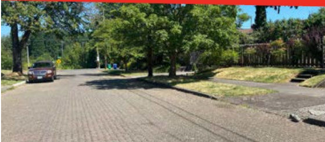
A Street paved with asphalt (top) and pavers (below) Portland, OR
