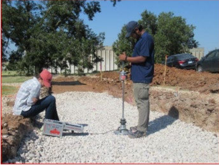
LWD Testing after 3 rd Lift (Zorn)
