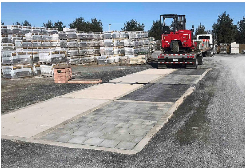
Test pad with slabs and planks on concrete and aggregate bases subject to tractor-trailer loads.
