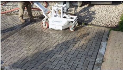
High pressure air and vacuum system
