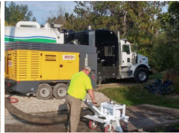
High pressure air and vacuum system
