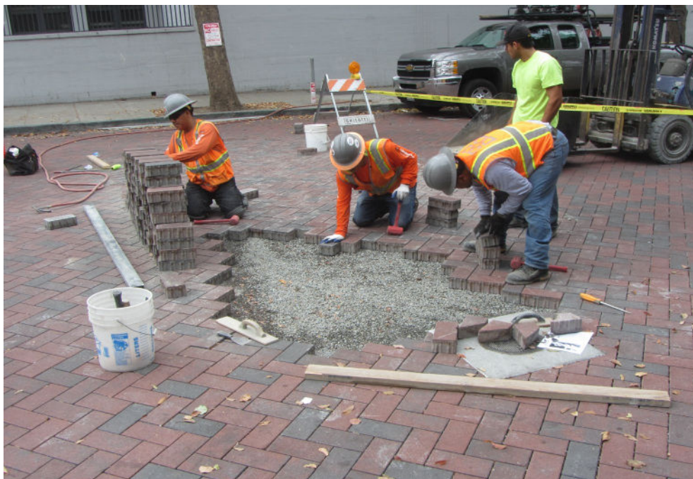
Figure 1-3. Utility Cut Repair of Interlocking Concrete Pavement.
