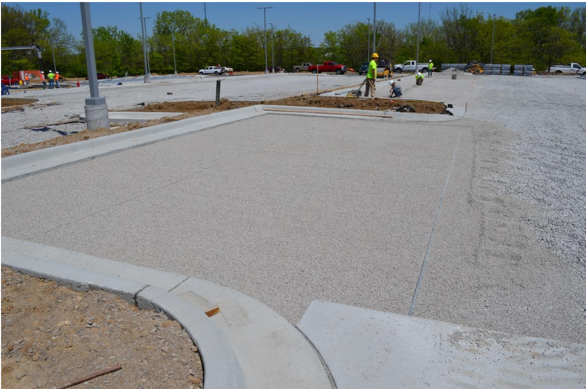
Figure 38. Final Grading of the Bedding Layer
