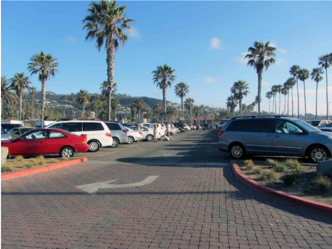
Figure 108. Photo of Example 2 PICP Parking Lot in La Jolla, CA (ICPI, 2015)
