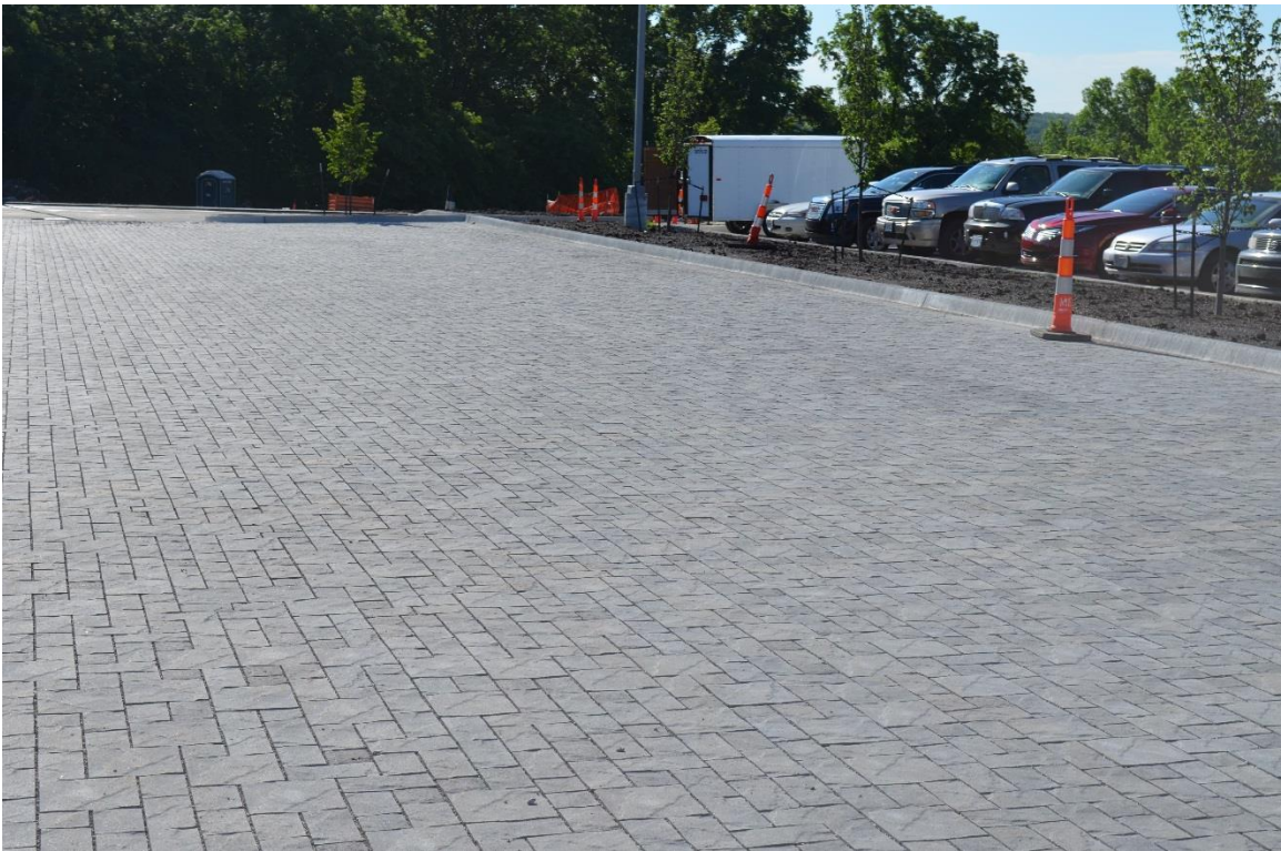
Figure 40. The Finished Installation after Compaction and Prior to Opening
