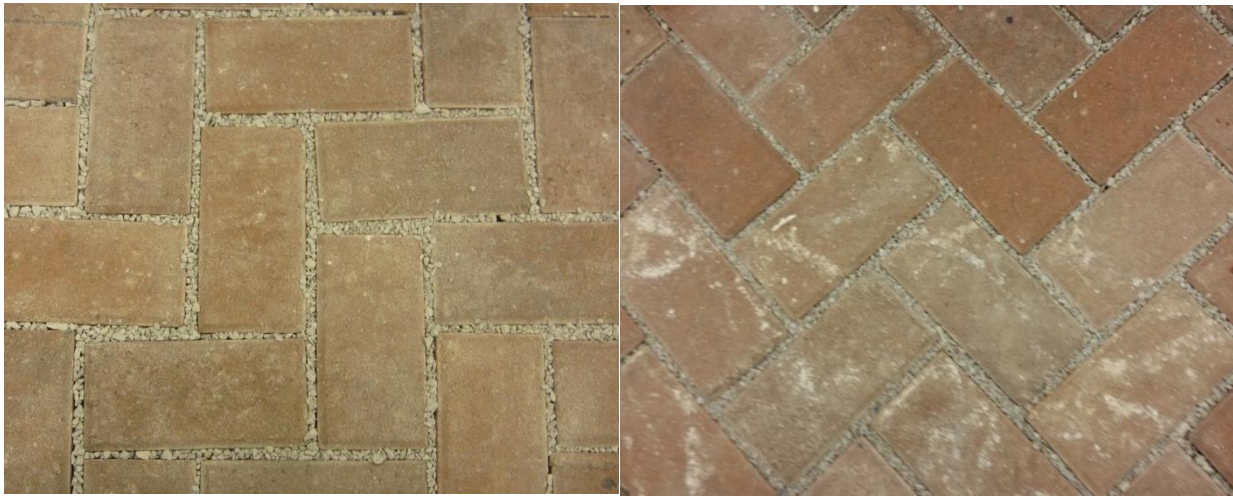
Figure 49. (Left) Straight herringbone Pattern 6 mm Spacing (right) 45 Degree Herringbone Pattern 6 mm Spacing
