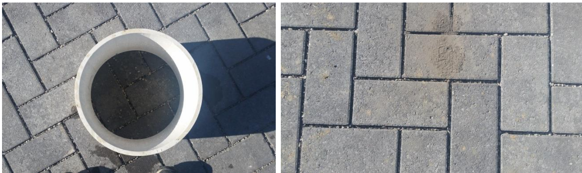
Figure 41. Water Services Vertical Test and Pavement 6 mm Straight herringbone
