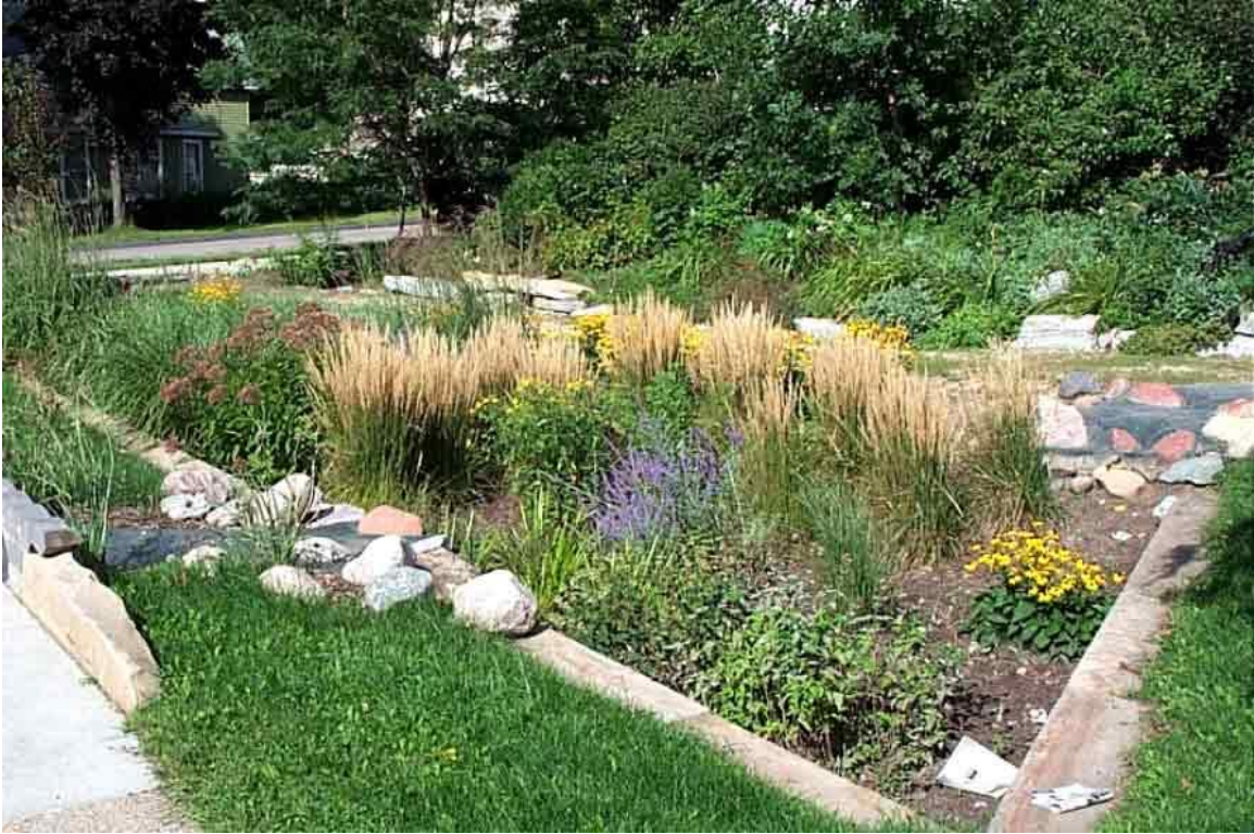
Figure 3. Examples of Structural BMP – Rain Garden (SUNY-ESF, 2015)
