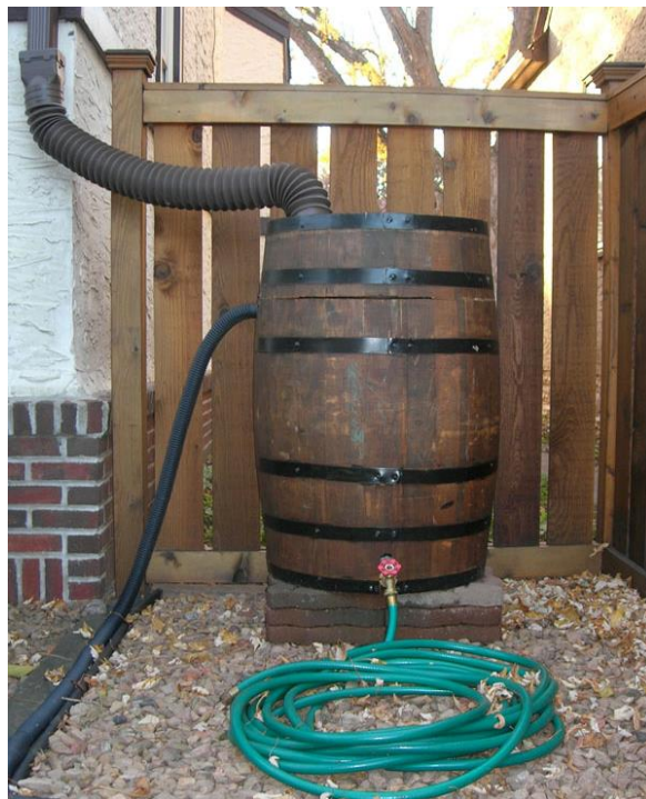
Figure 4. Example of Structural BMP - Rain Barrel (Rutgers, 2014)
