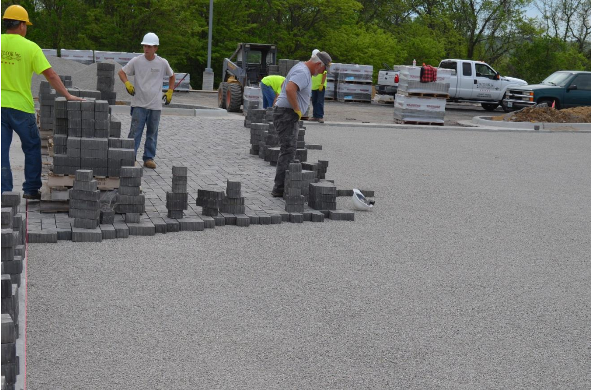
Figure 39. Setting the Straight Herringbone Pattern By Hand
