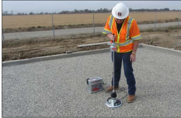
Figure 5.13: Light-weight deflectometer testing on the base.
