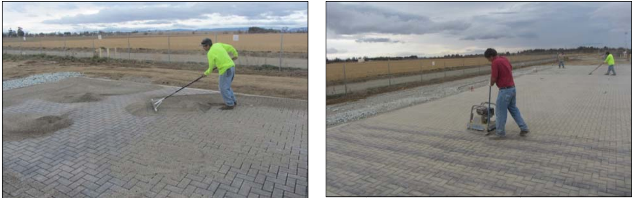
Figure 5.16: Jointing stone placement and compaction.
