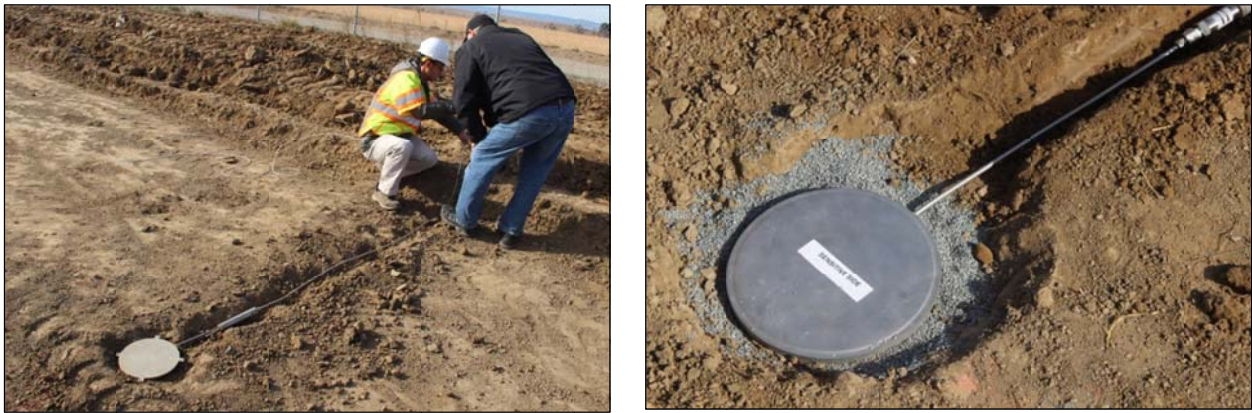
Figure 6.10: Pressure cell installation in the subgrade.
