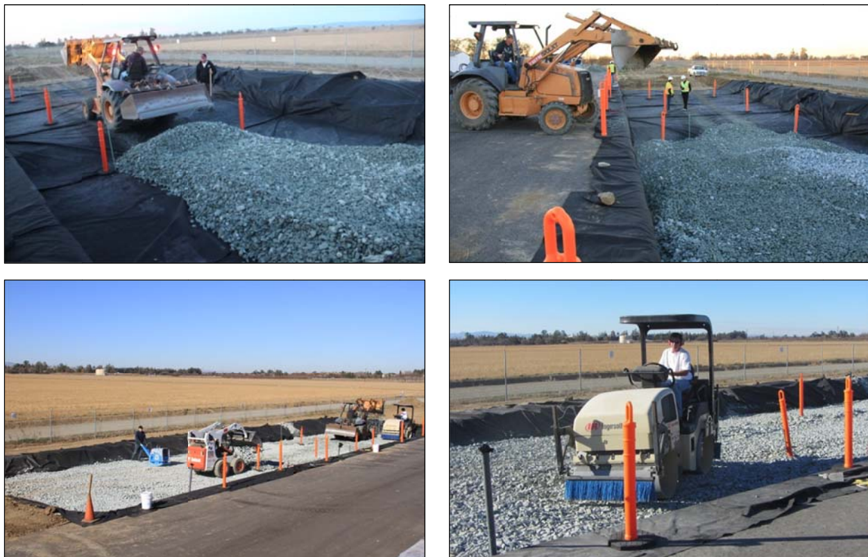
Figure 5.8: Placing and compacting the subbase.
