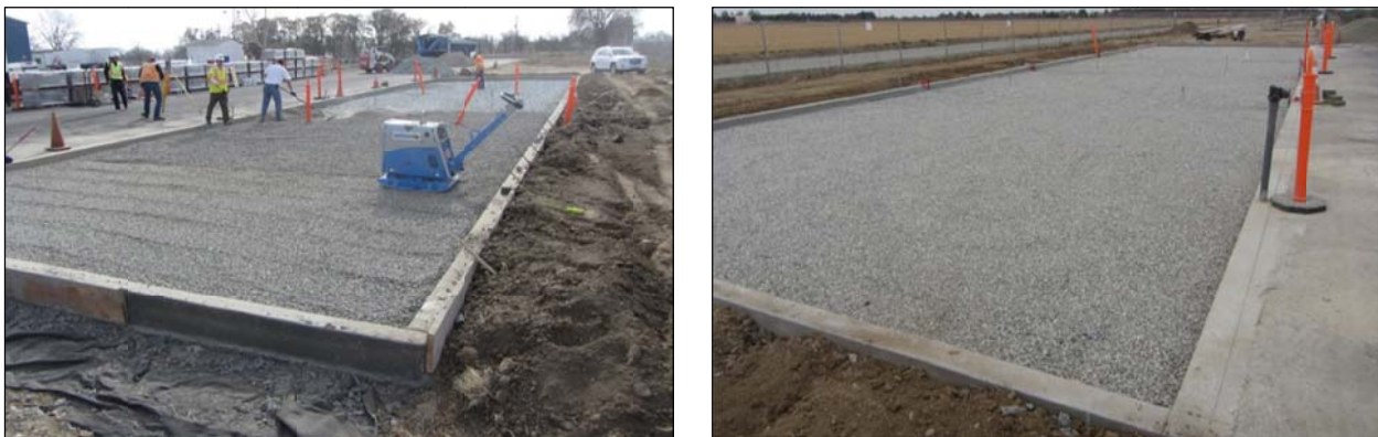
Figure 5.12: Base layer placement.
