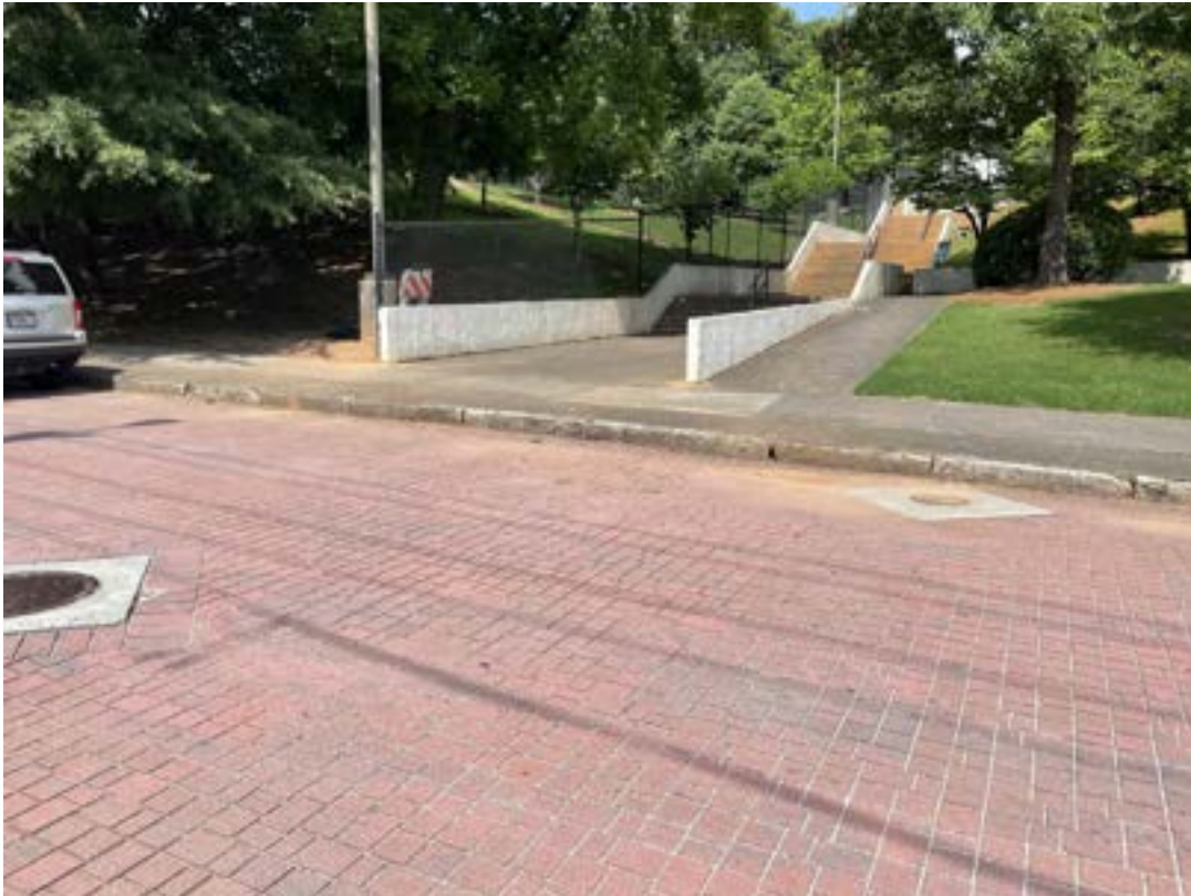
Pavers on a street in Atlanta, GA
