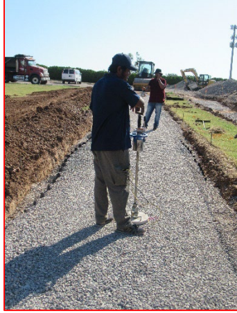
LWD Testing on Geo-cell Reinforced Section (Olson)
