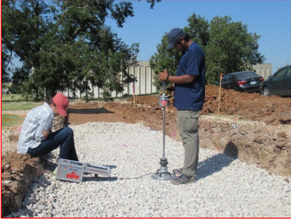
LWD Testing after 3 rd Lift (Zorn)
