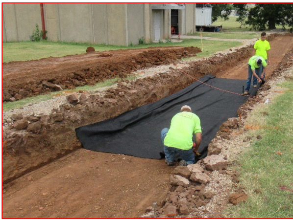
Geotextile Placement
