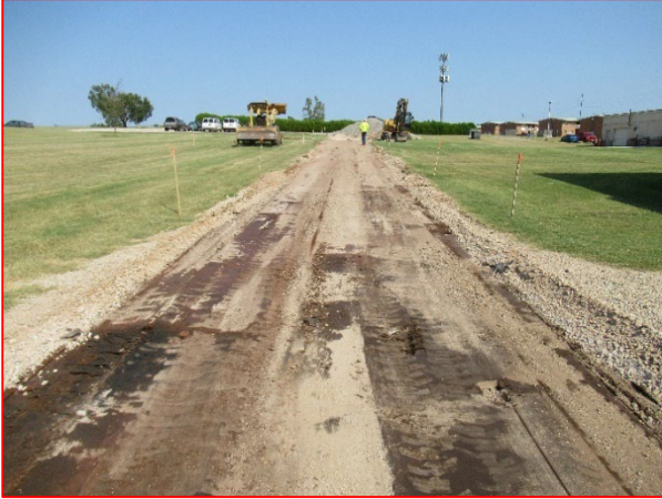
Unprepared Subgrade
