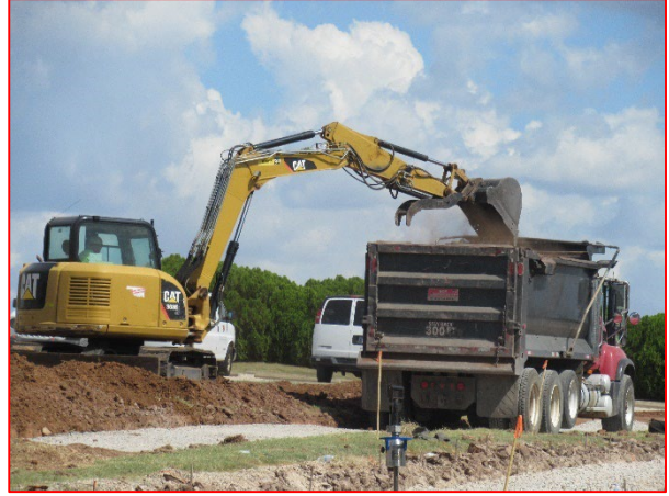
Transportation of the Excavated Soil
