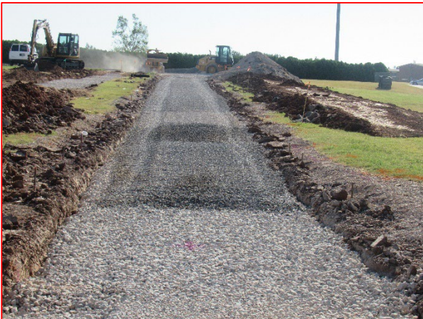
Placement of 4 th Lift (4in ASTM#4)
