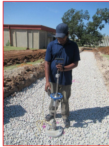
LWD Testing after 3 rd Lift (Olson)
