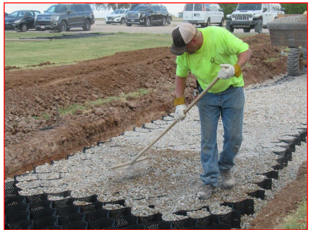
Leveling the Top Surface of the Geo-Cell
