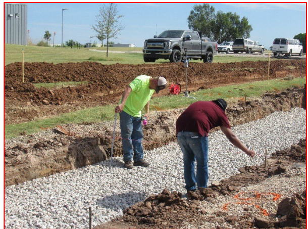
Aggregate Placement and Depth Check
