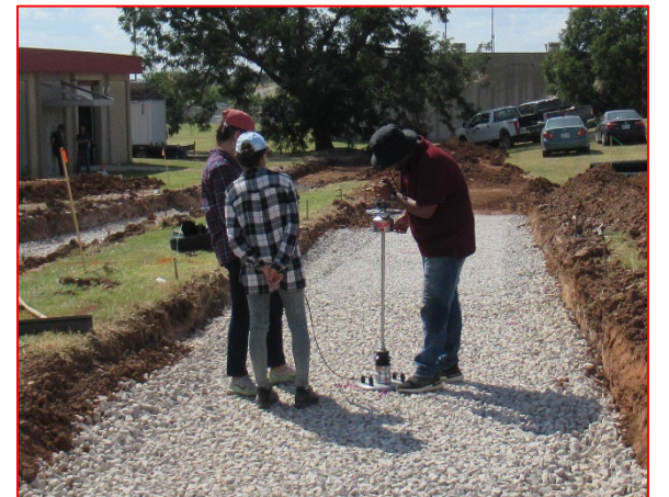
LWD Testing after 2 nd Lift (Olson)
