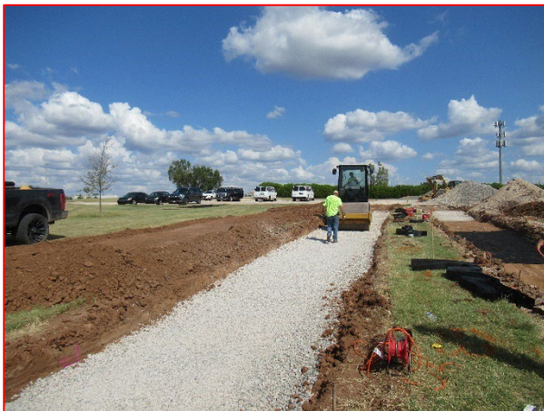
Compaction After 2 nd 6in Lift
