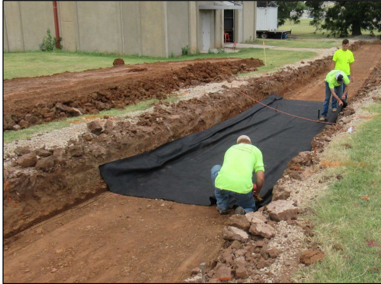
Figure 29: Photograph Showing Geotextile Placement at the Subgrade-Subbase Interface
