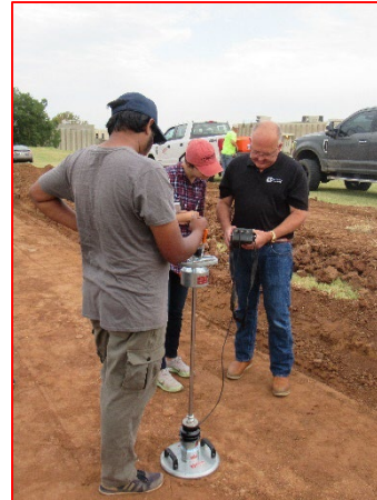
Zorn LWD Testing on Subgrade
