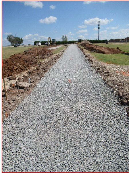
Finished Subbase and Base
