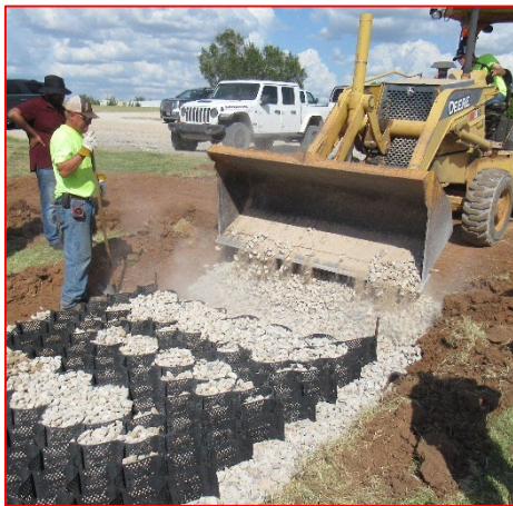
Placing Aggregate into the Geo-cell
