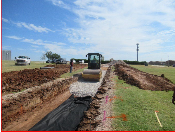
Compaction of 1 st 4in Lift
