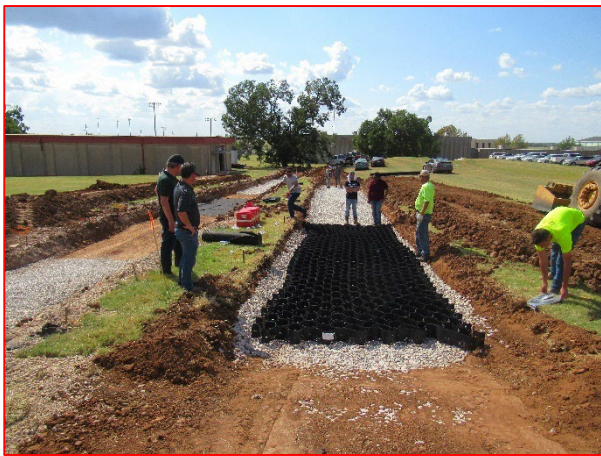
Geo-Cell Placement on Top of 2in Aggregate Material
