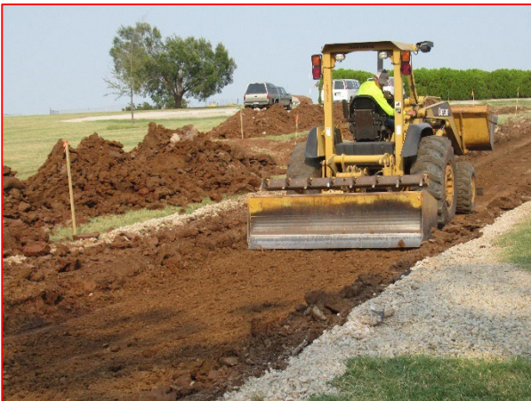
Leveling of Soil by Backhoe Loader
