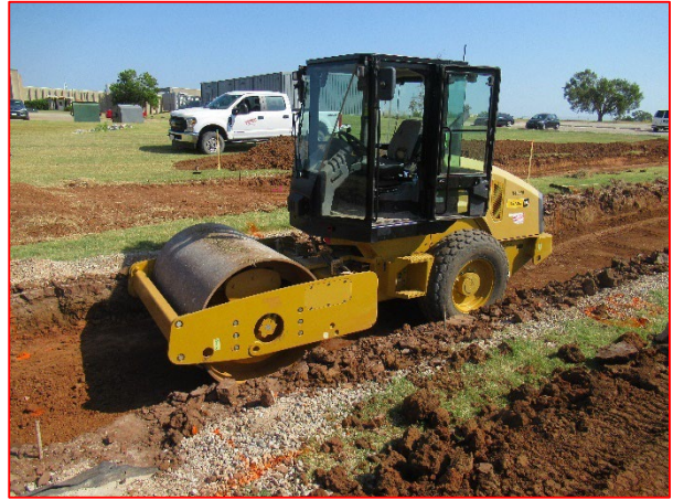
Compacting Subgrade
