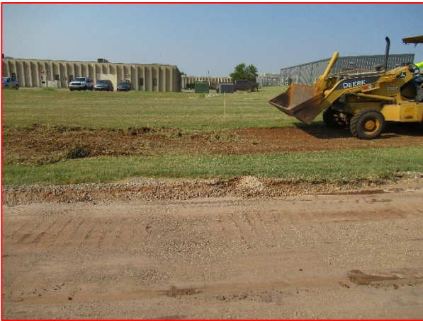
Removal of Grass, Weeds
