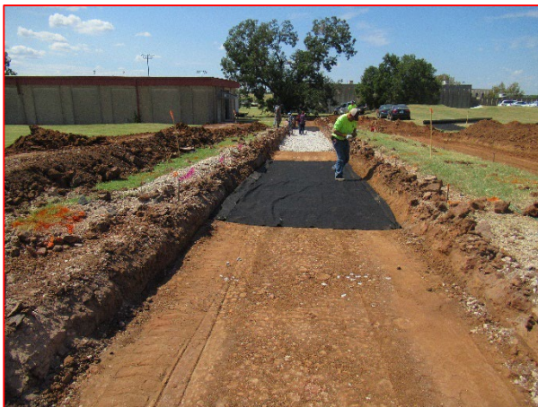
Preparing Other Test cells for Aggregate Placement
