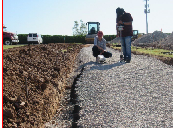
LWD Testing on Geo-cell Reinforced Section (Zorn)
