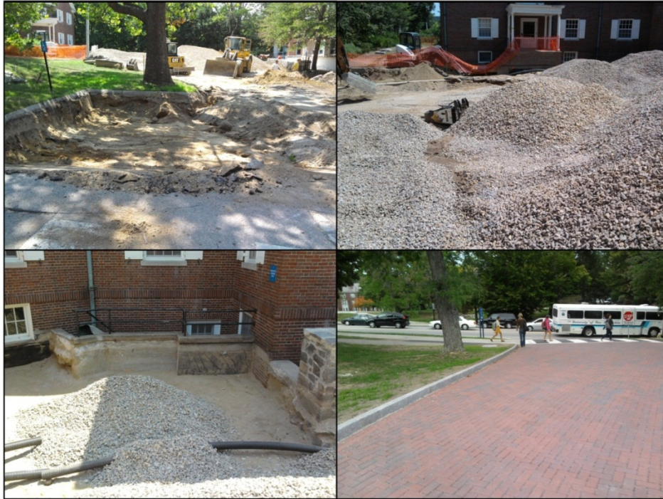
Figure 1: August 2010 installation of PICP system (clockwise from top left) demolition and excavation, placement of subbase aggregate, finished product, underdrain installation.
