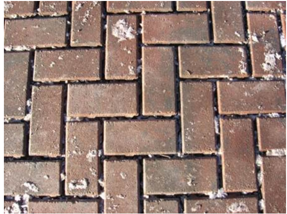
Figure 15: No. 8 joint stone has settled approximately 1 inch.
