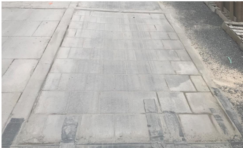
Figure 5: Cell 3. 12 x 12 x 3.125 in. thick units on an aggregate base.
