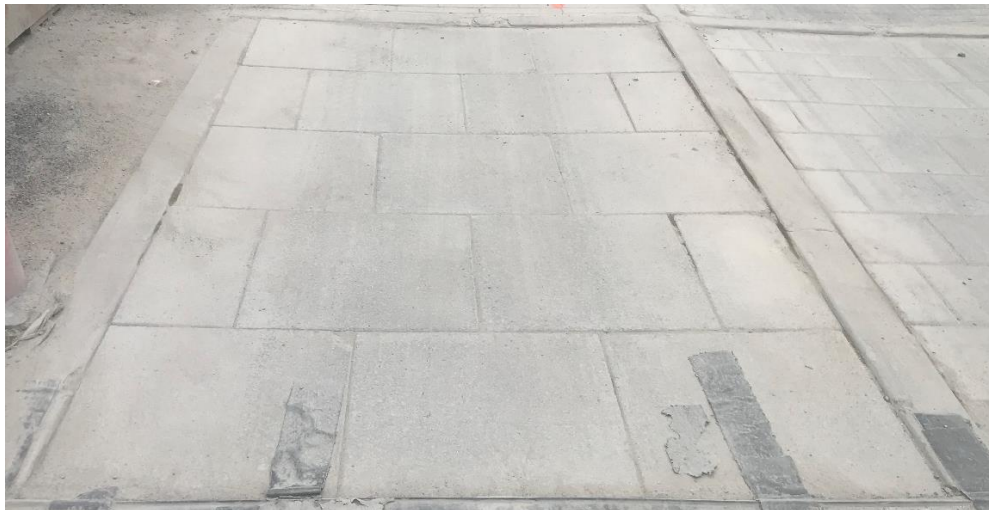
Figure 9: Cell 7. 24 x 24 x 3.125 in. thick units on an aggregate base.
