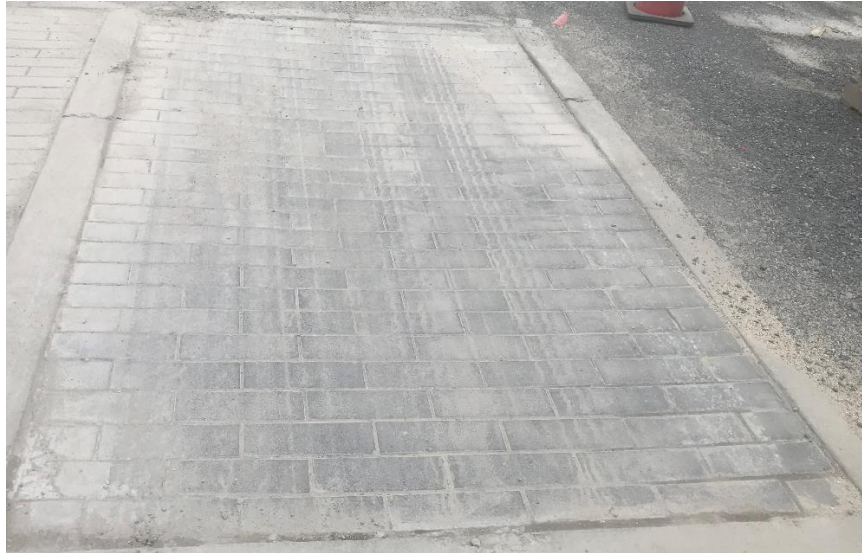
Figure 6: Cell 4. 4 x 12 x 4 in. thick units on an aggregate base.
