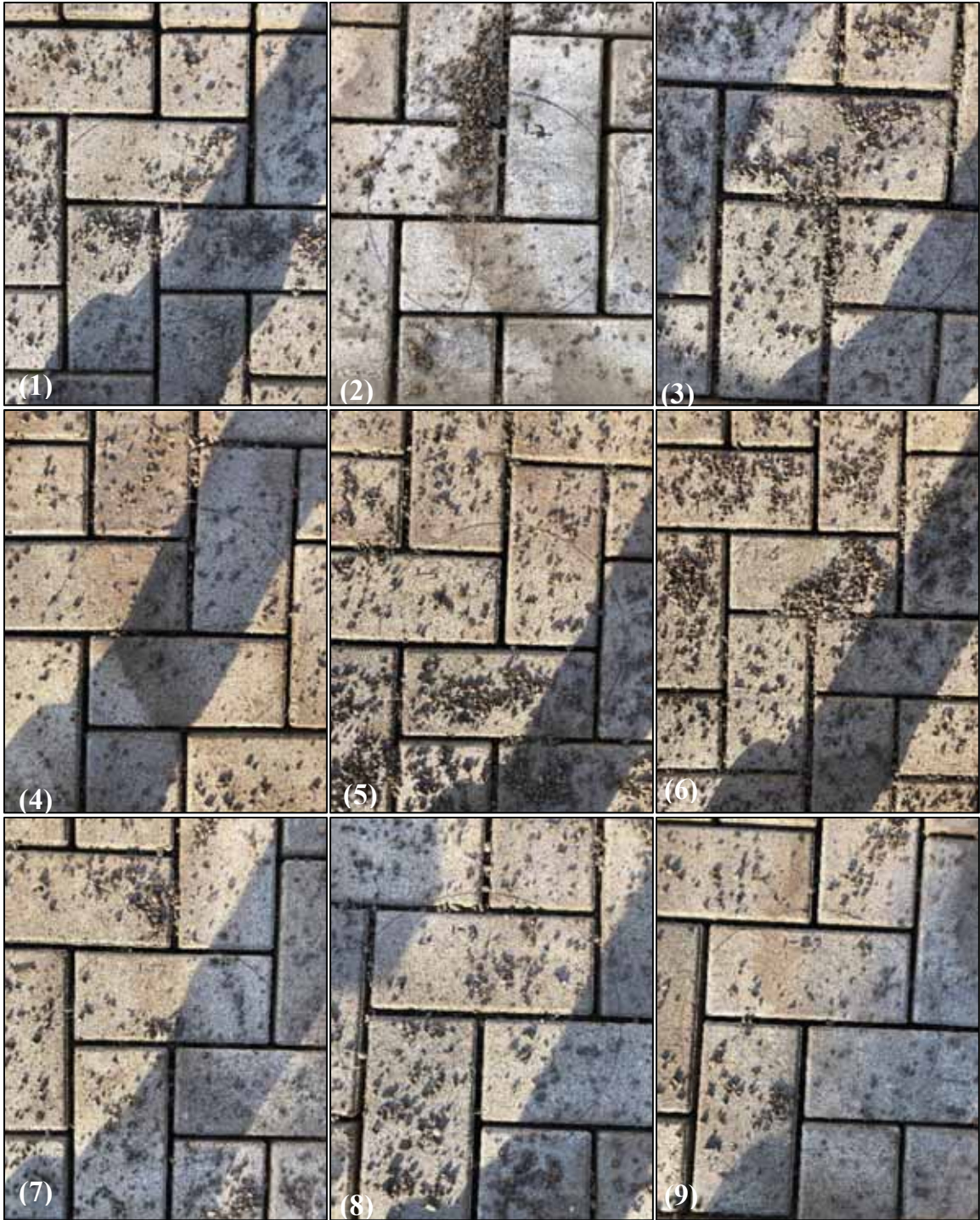
Figure I2: Post-maintenance photos of infiltration measurement locations (1-9) following high pressurized-air system on Cell 1 (Pave-Tech Typhoon®).
