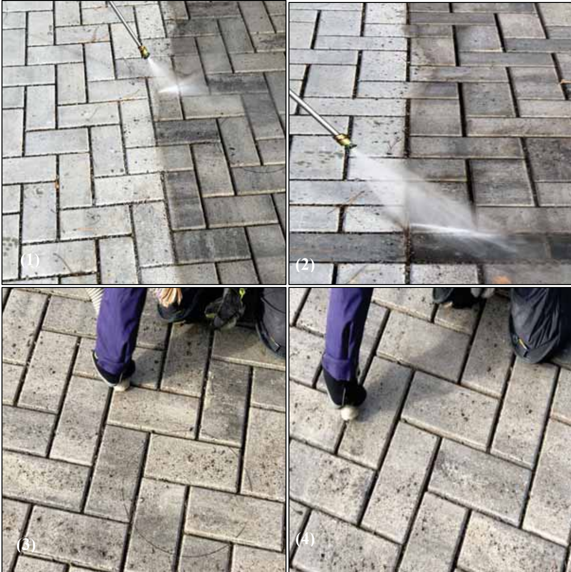
Figure I5. Pre- and post-maintenance following pressure washing (1,2) and vacuuming (3,4) on Cell 3.
