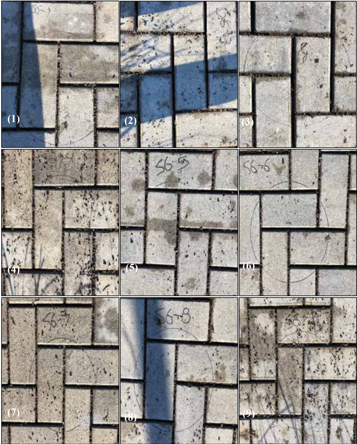
Figure J2. Post-maintenance photos of infiltration measurement locations (1-9) following a regenerative air street sweeper on Cell 6 for first early and repeated maintenance (TYMCO DST-6®).
