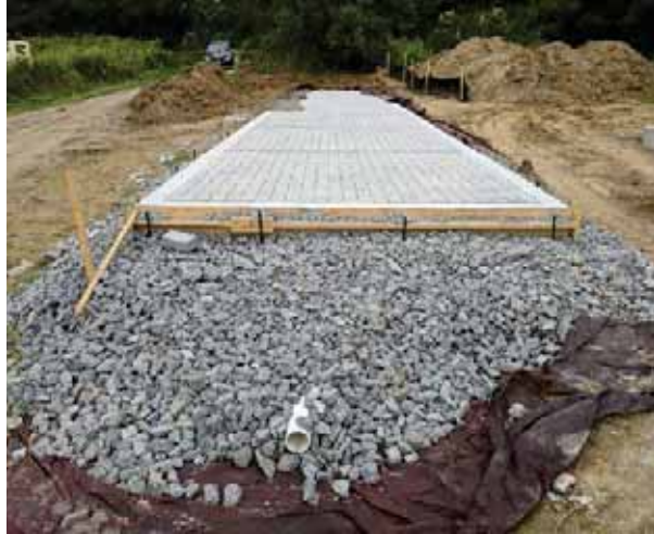
Figure 2-2: Test pad following construction (Aug 18 th , 2017).
