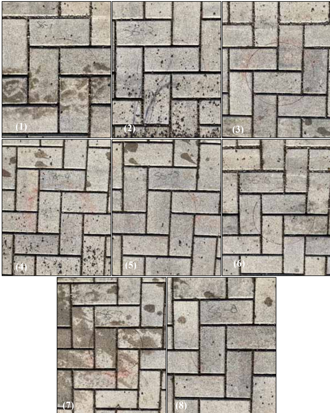
Figure J6. Post-maintenance photos of infiltration measurement locations (1-8) following a regenerative air street sweeper on Cell 6 for third early and repeated maintenance (TYMCO DST-6®).
