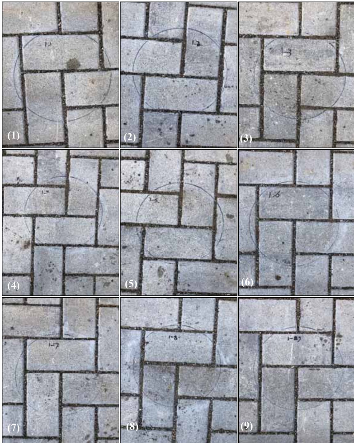
Figure I1: Pre-maintenance photos of infiltration measurement locations (1-9) on Cell 1 (Pave-Tech Typhoon® and Pavevac®).
