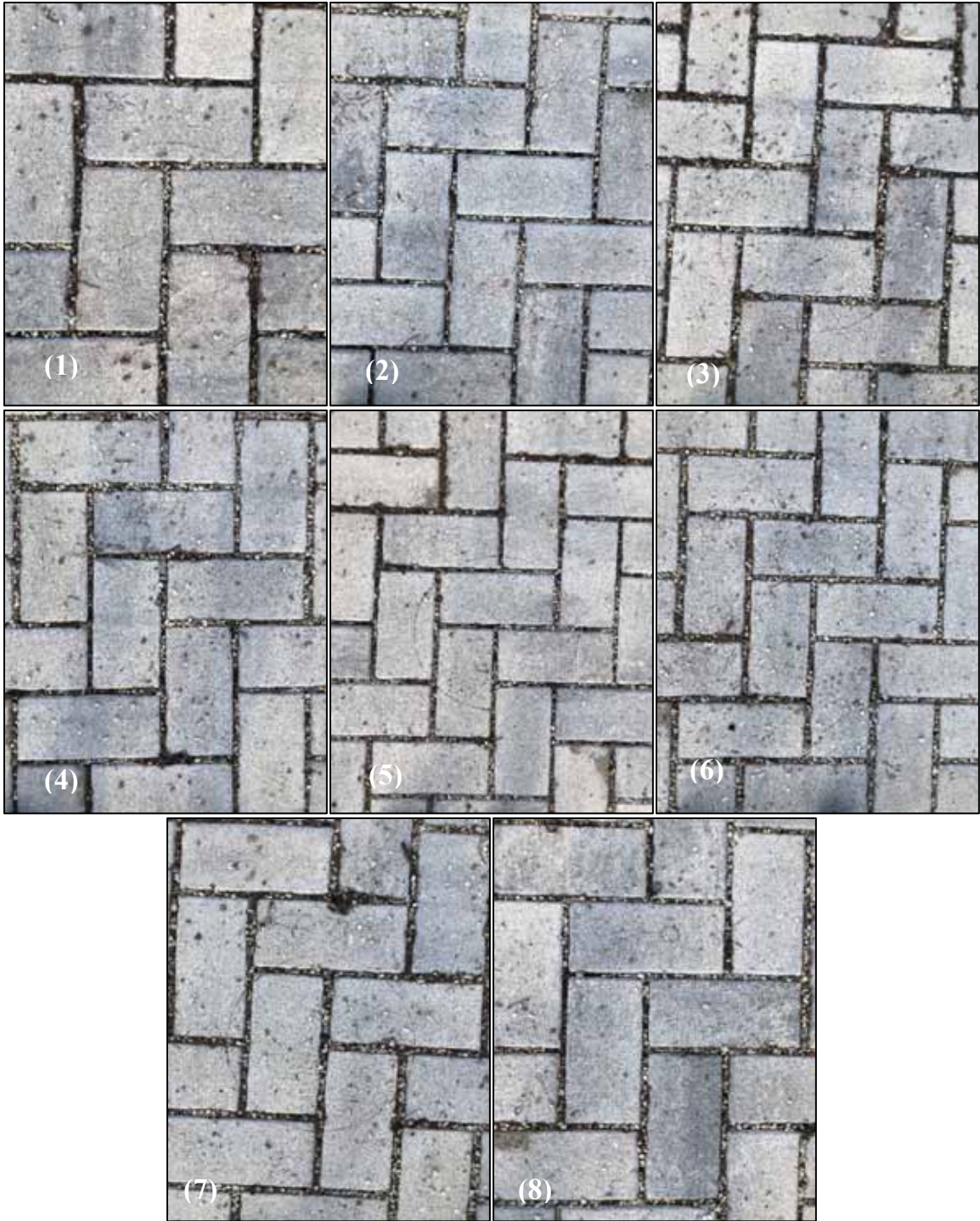
Figure J7. Pre-maintenance photos of infiltration measurement locations (1-8) on Cell 6 after third early and repeated maintenance (TYMCO DST-6®).
