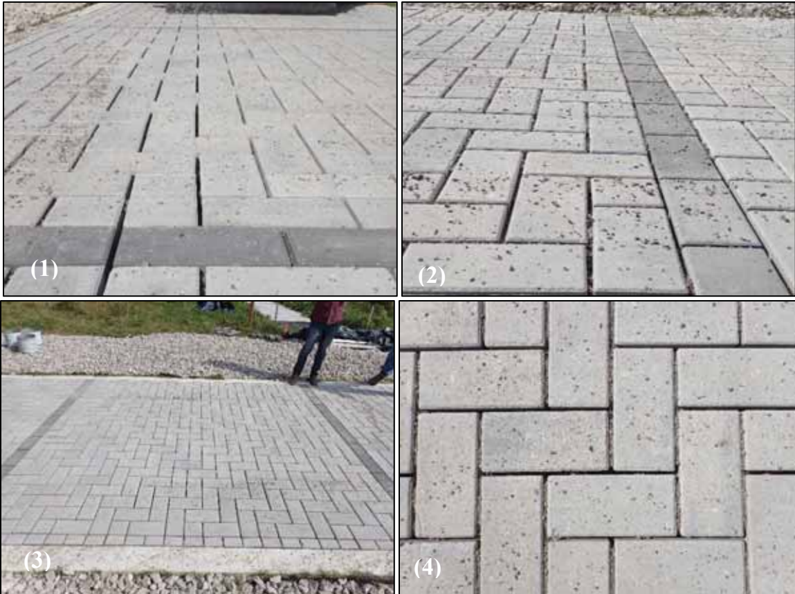
Figure 17. Post maintenance photos following a waterless mechanical sweeper on Cell 5 (Elgin Sweepers Water Less Eagle ® ), where (1) and (2) are parallel and perpendicular to travel path respectively. (3) is an overview of the plot and (4) is a close up of parallel and perpendicular sediment removal.
