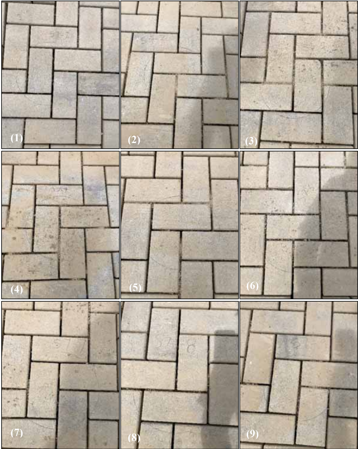
Figure K3. Post-maintenance photos of infiltration measurement locations (1-9) following a vacuum system on Cell 7 (Pavevac®).
