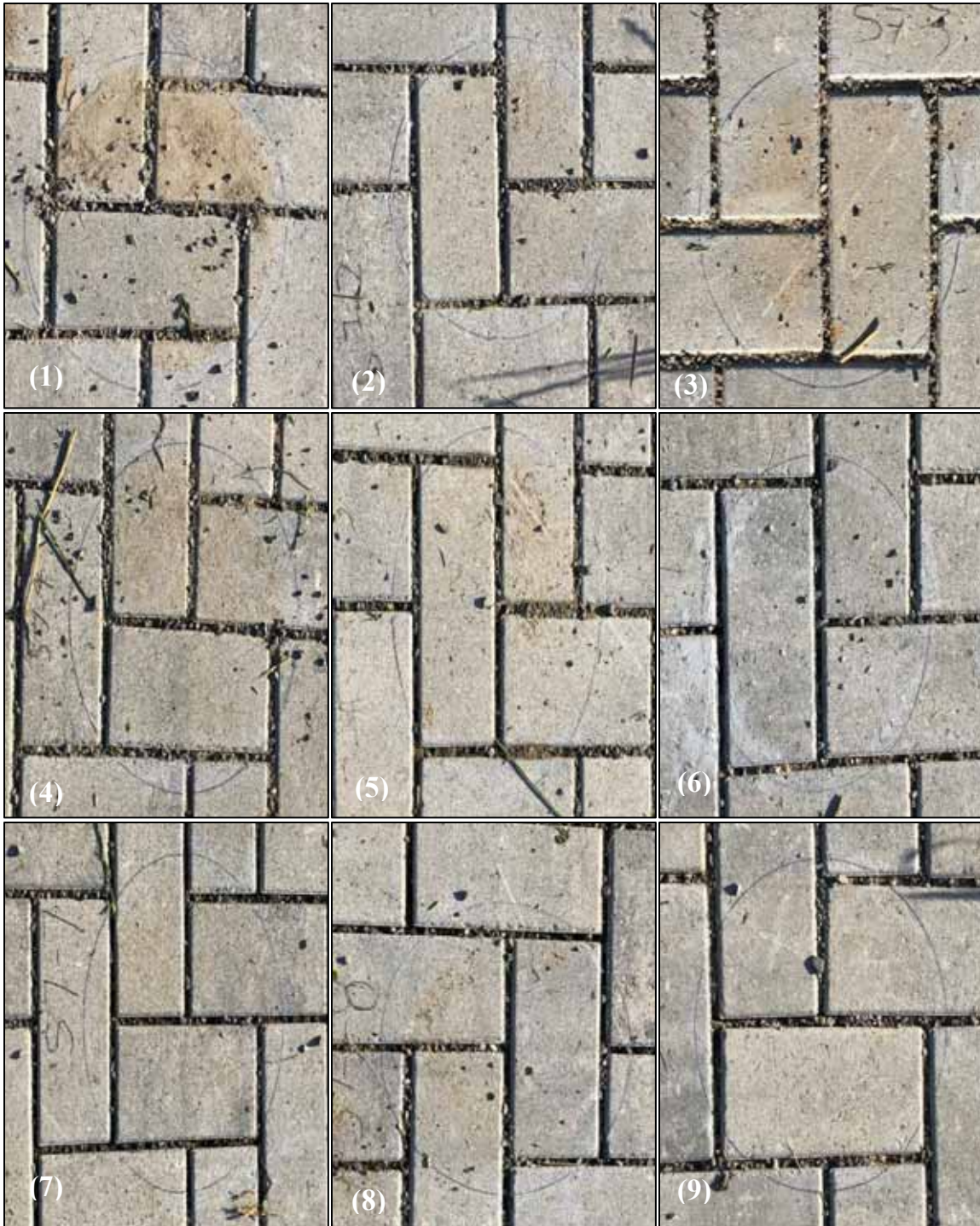
Figure K1. Pre-maintenance photos of infiltration measurement locations (1-9) on Cell 7 (Pave-Tech Typhoon® and Pavevac®).
