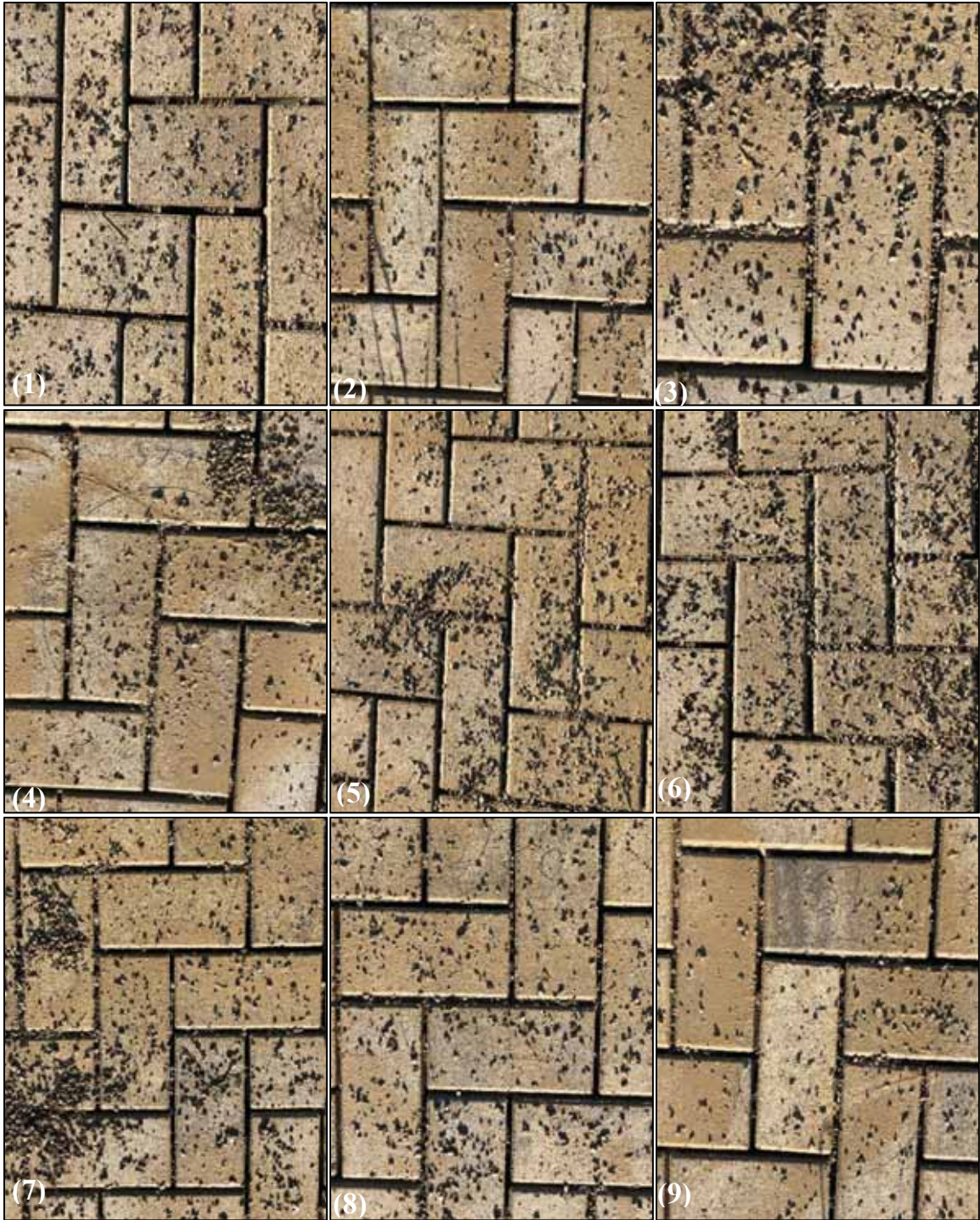
Figure K2. Post-maintenance photos of infiltration measurement locations (1-9) following high pressurized-air system on Cell 7 (Pave-Tech Typhoon®).
