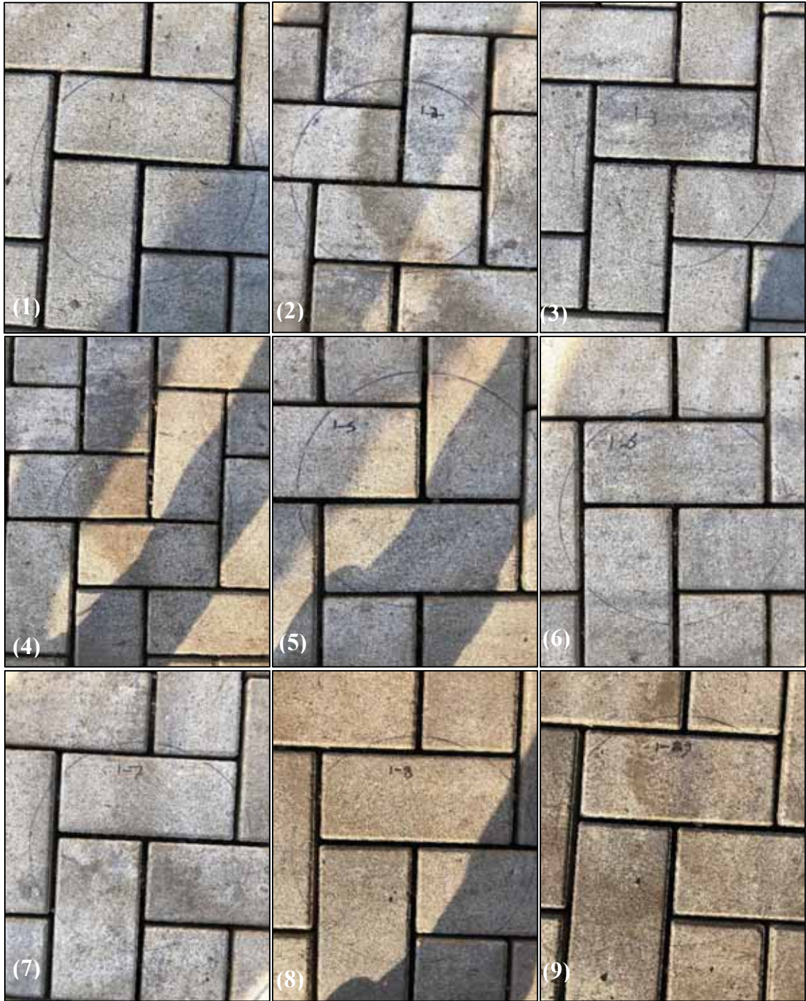
Figure I3. Post-maintenance photos of infiltration measurement locations (1-9) following a vacuum system on Cell 1 (Pavevac®).
