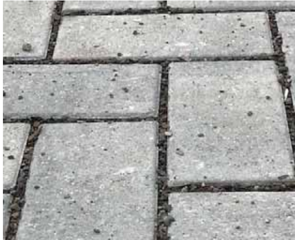
Figure 3-5: Visual inspection of the PICP joints after the third round of clogging before compaction
