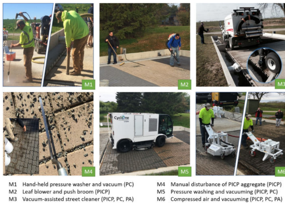
Figure 5. Images of the six different maintenance practices that were evaluated for use on permeable interlocking pavers (PICP), pervious concrete (PC), and porous asphalt (PA) test plots.
