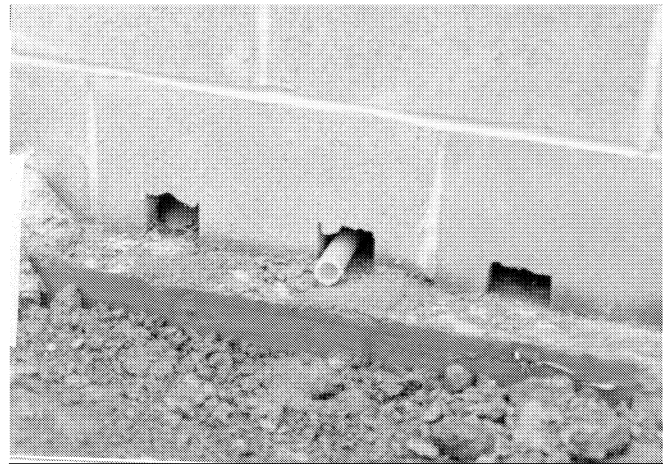
Figure 4-7: Weep Holes At The Base Of A Foundation
