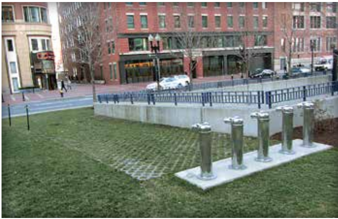
Figure 7. Emergency access lane for fire trucks
