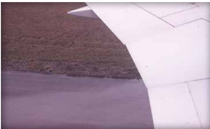
Figure 11. Airfield taxiway shoulder
