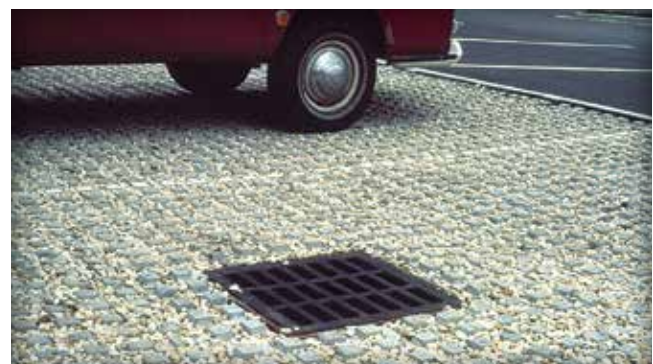
Figure 16. Concrete grids with aggregate in the openings
