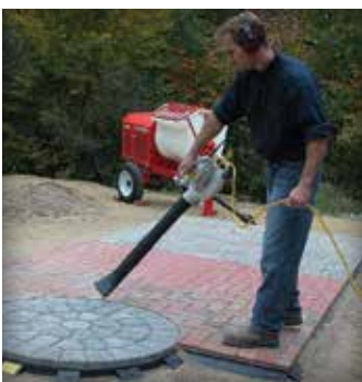
Figure 6. Whether using liquid or dry joint stabilization materials, the surface of the pavers should be cleaned with a blower or broom after the joint sand is compacted into the joints.
