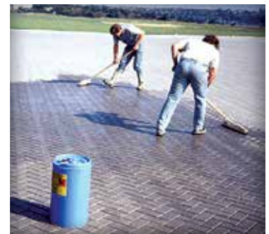
Figure 10. Urethane is applied with squeegees to stabilize joint sand between pavers on aircraft pavement.
