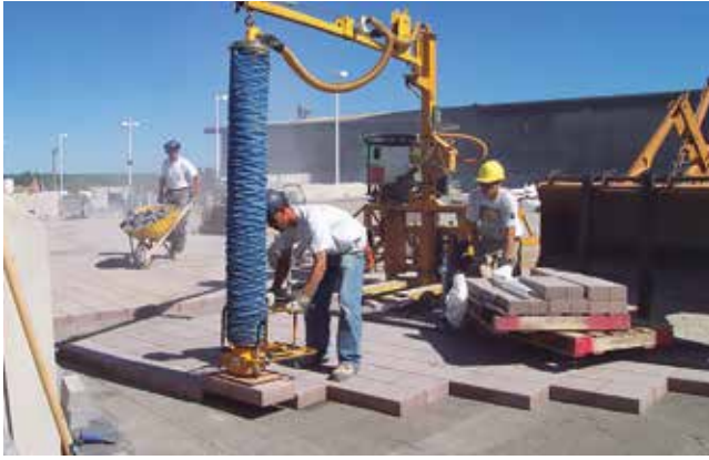
Figure 12. Self-contained vacuum lifter with boom
