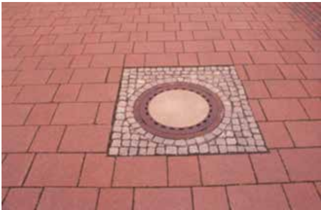
Figure 29. Filling the outside of a utility cover with mortar-set stone paving units
