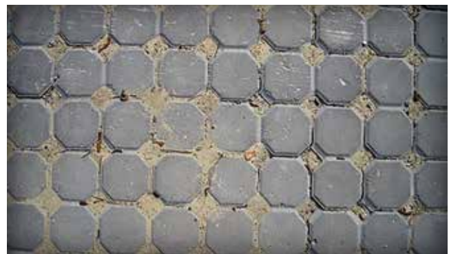
Figure 6. Sand from winter maintenance must be removed the following spring.
