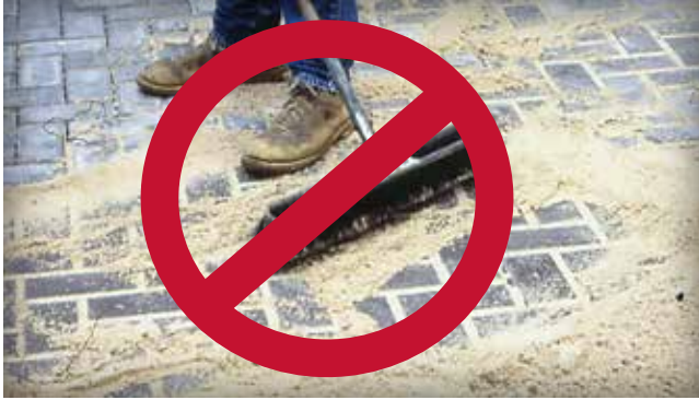
Figure 2. Sand-filled joints and bedding common to interlocking concrete pavement are not used in PICP.
