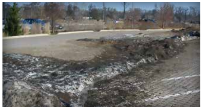
Figure 26. This is an example of snow that should have been deposited on a grassy area. If such areas are not available, then vacuum clean the PICP in the early spring.
