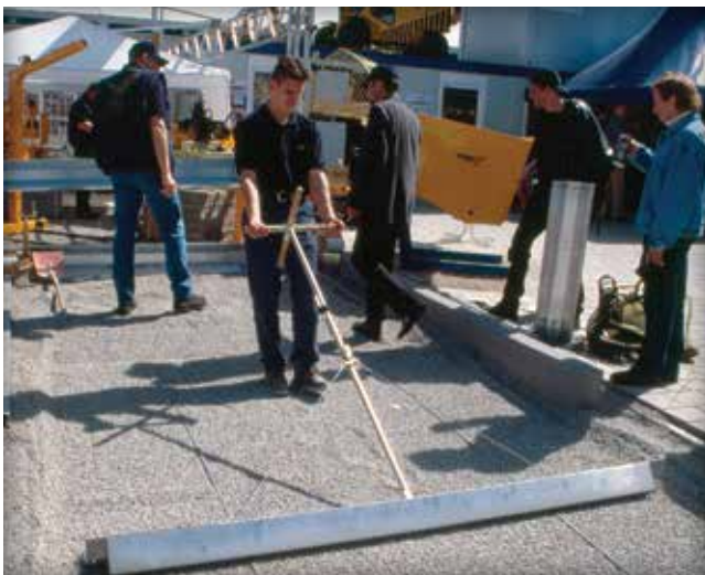
Figure 24. Manually screeding the No. 8 stone setting bed.
