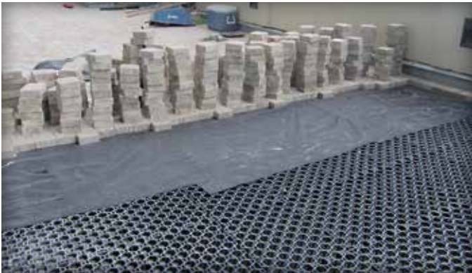
Figure 7. Concrete pavers on geotextile over plastic grids
