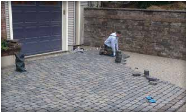
Figure 11. Concrete pavers installed to accommodate permeable bedding and jointing materials, all supported by a permeable stone base.
