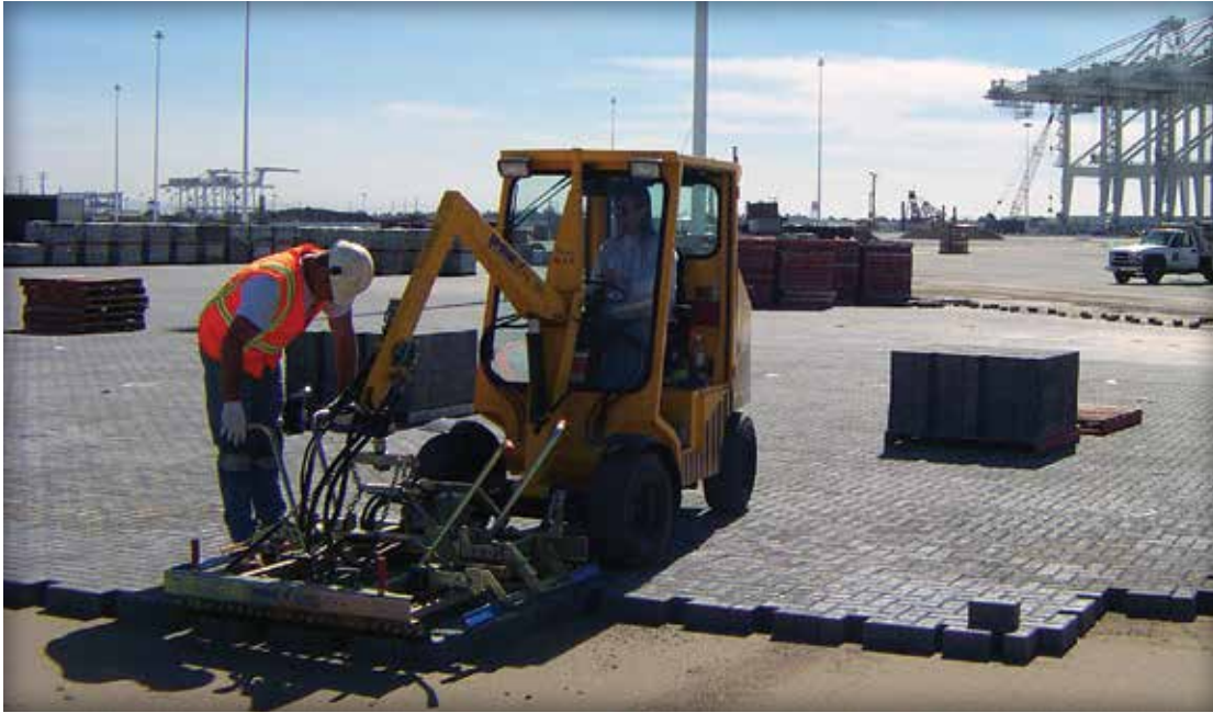
Figure 8. Mechanical installation equipment places concrete pavers rapidly.
