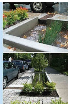
SW 12th Avenue Green Street Project Portland, Oregon Kevin Robert Perry, ASLA
