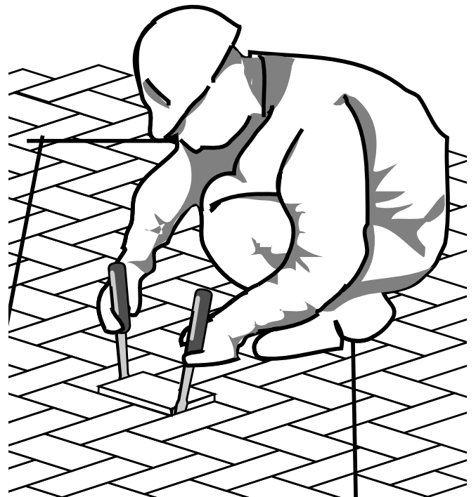
Figure 31. A pair of slot screwdrivers can also be used to wiggle out the first paver. Care must be used to slowly work the unit out and not damage the surround paver edges.
