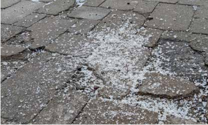
Figure 8. Use deicing chemicals sparingly and remove any excess after it has completed its job.
