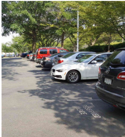
Before: asphalt pavement
