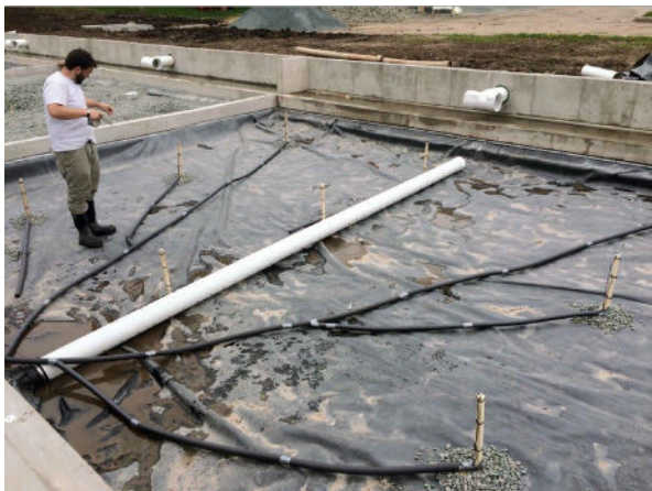
Installation of temperature sensors.
