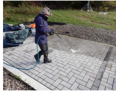
Power washing before applying a Shop Vac
