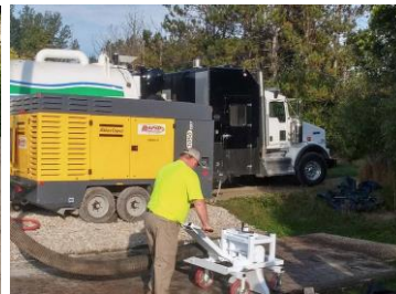
High pressure air and vacuum system
