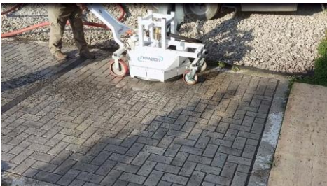
High pressure air and vacuum system
