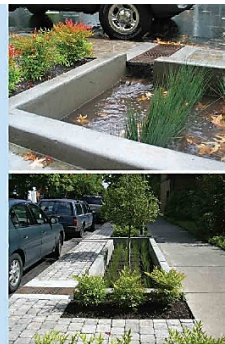
SW 12th Avenue Green Street Project Portland, Oregon Kevin Robert Perry, ASLA
