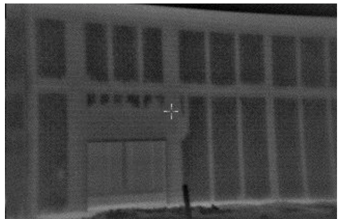
Figure 3—Infrared Photograph Used to Verify Proper Grout Placement
