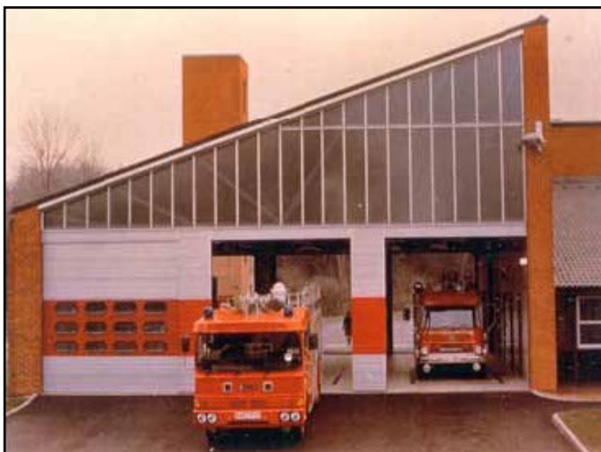
Figure 1—Fire Station With Diaphragm Wall (courtesy of Malcolm Phipps)
