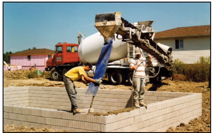
Figure 4— A Residential, Mortarless, Single-Family Basement - Part of a 520 Home Development
