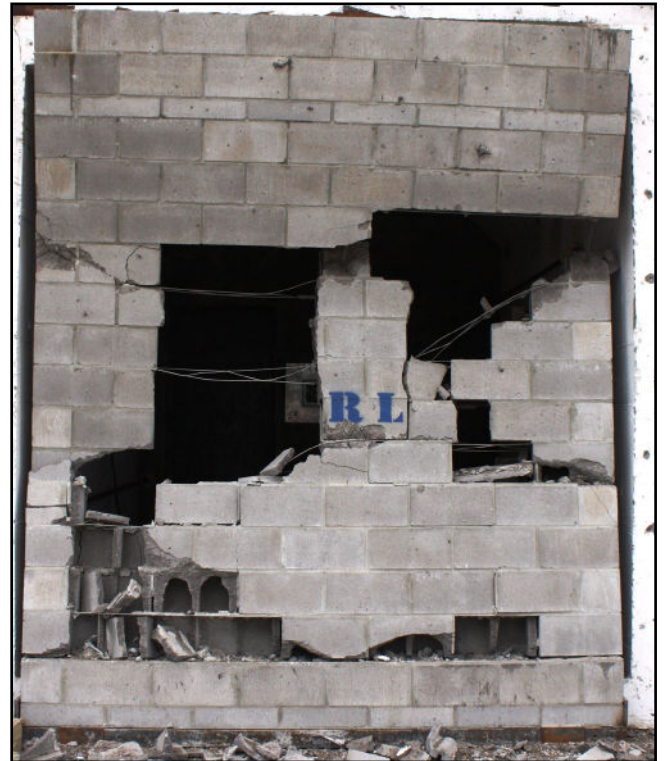
Figure 2—Result of Full-Scale Explosion Testing of Partially Grouted CMU Demonstrating Breaching Tendency
