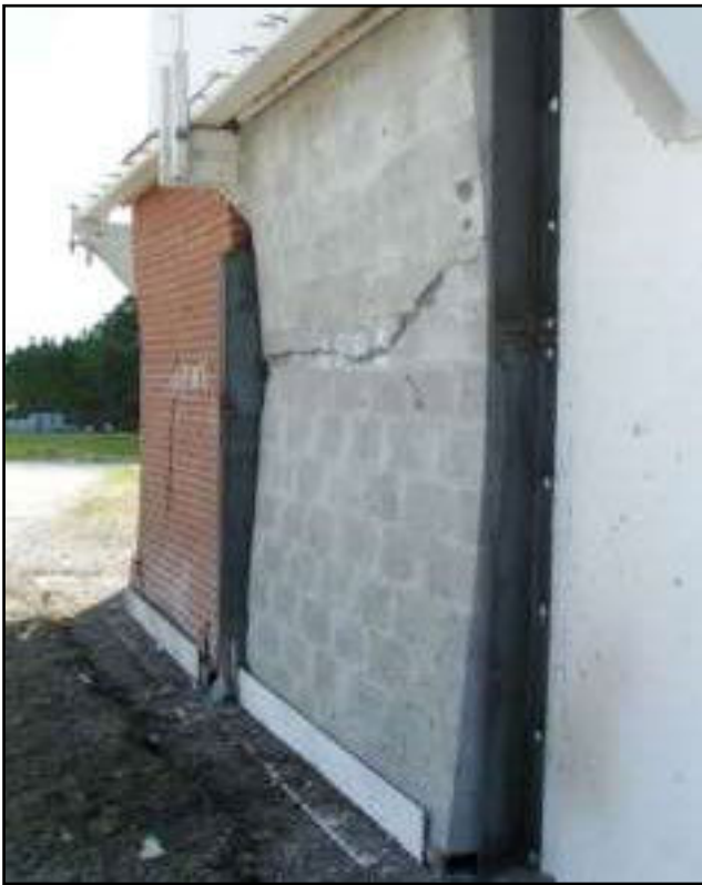
Figure 1—Result of Full-Scale Explosion Testing of Fully Grouted CMU and Cavity Walls
