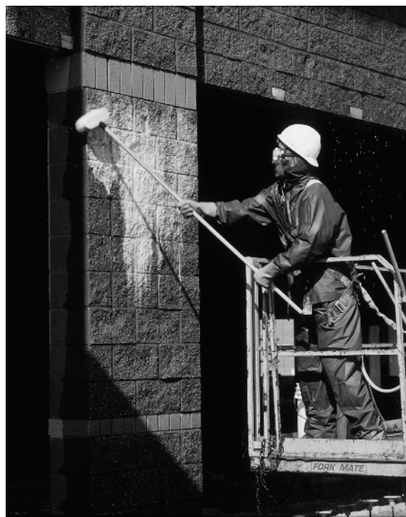
Figure 1—Pressure Chemical Cleaning (photo courtesy of PROSOCO, Inc.)
