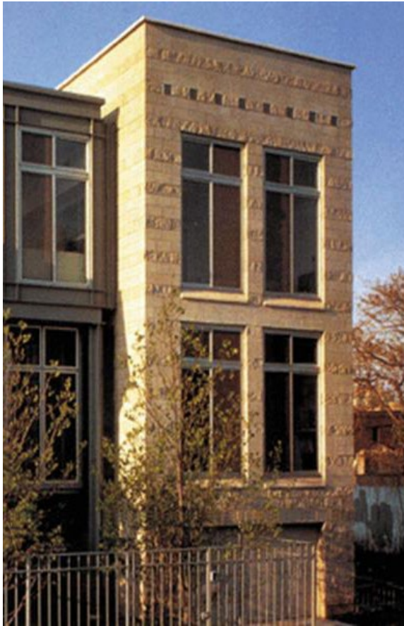
Figure 5—Banding Example: Split-Faced Bands in Ground Face Field
