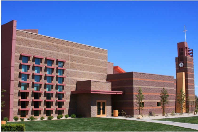
Use of complementary mortar to emphasize pattern
