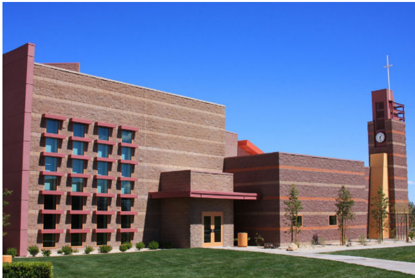
Use of complementary mortar to emphasize pattern
