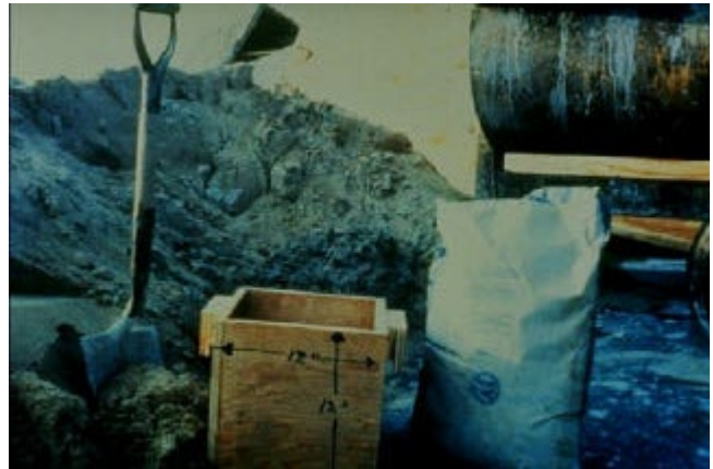
Figure 1—Measuring Mortar Sand Volume
