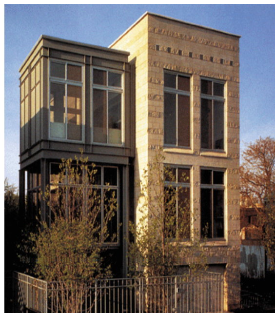
Figure 1—Exterior Concrete Masonry in a Residence
