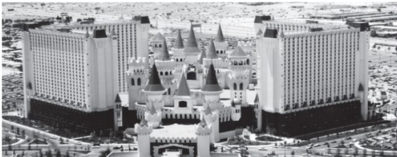
Figure 1—The four towers of the 28-story Excalibur Hotel in Las Vegas are load-bearing masonry.
