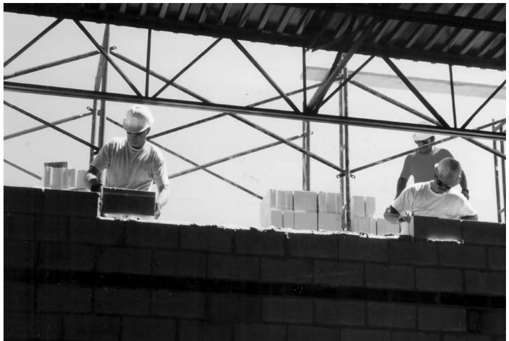
Placement of Concrete Masonry Units
