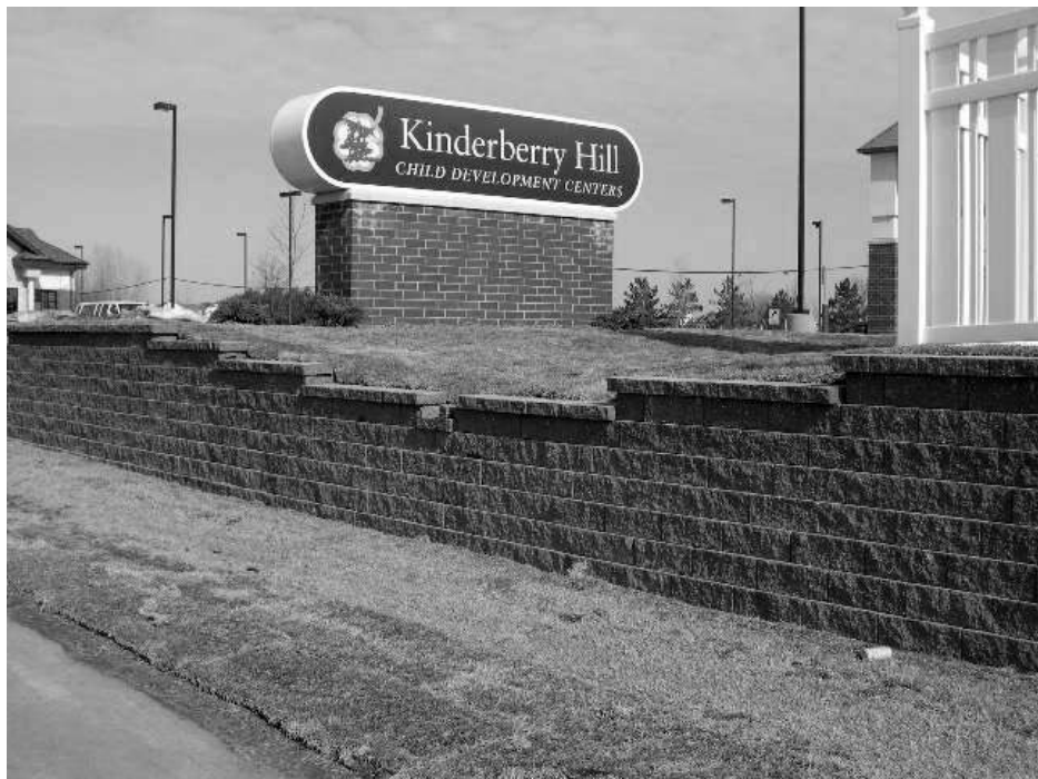
Figure 11-1: Surface Drainage Feature on a SRW
