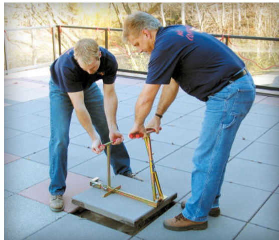
Figure 11. Double hand clamp for lifting larger paving slabs
