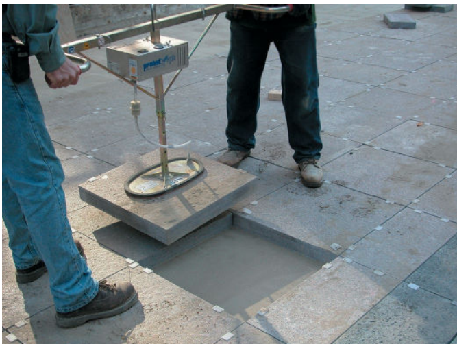
Figure 14. Two-person vacuum lift for paving slabs
