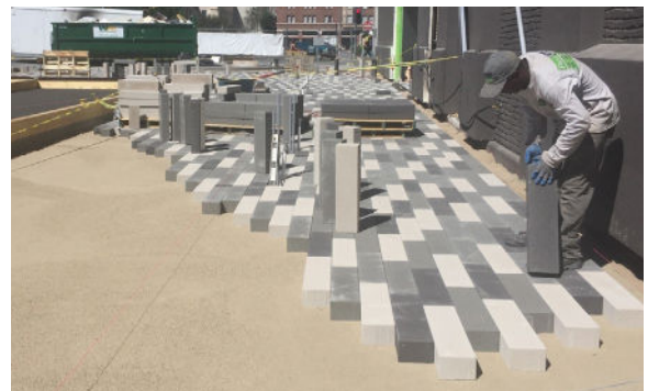
Figure 6. Installing planks on uncompacted bedding sand.
