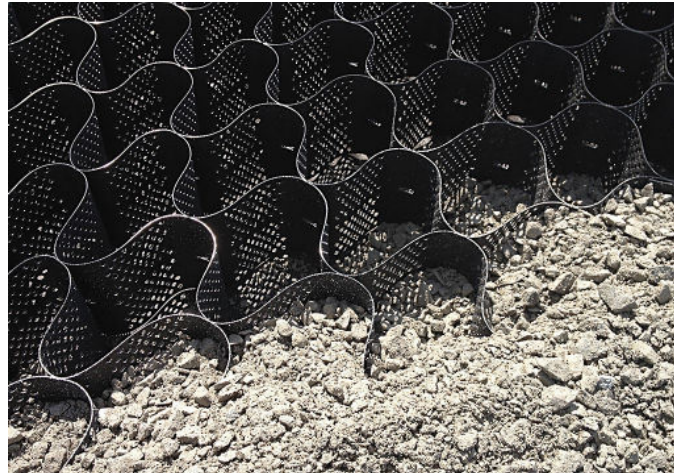
Figure 9. Geocells partly filled with aggregate
