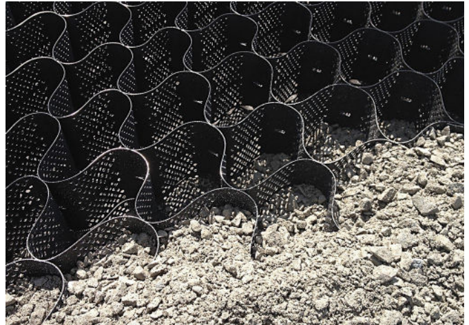
Figure 9. Geocells partly filled with aggregate
