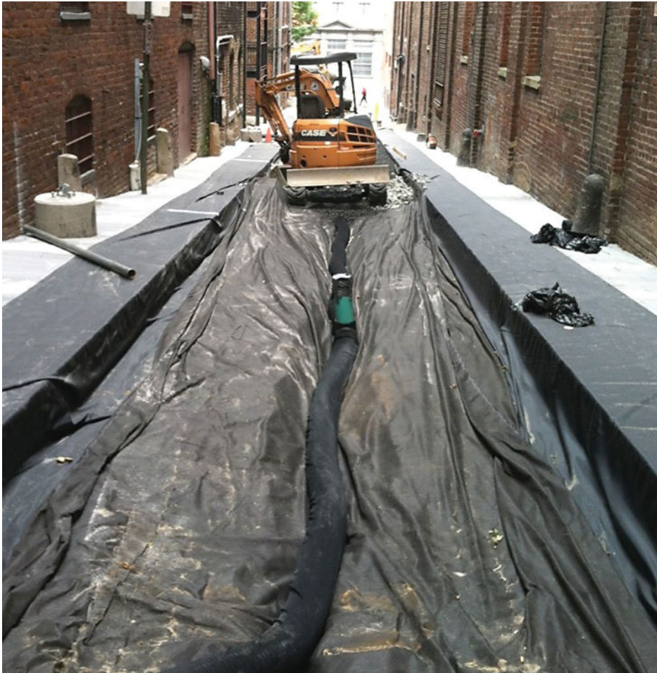
Figure 26. Geomembrane protected with a nonwoven geotextile for a PICP alley.
