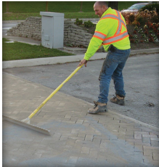
Figure 11. Sweeping in joint sand
