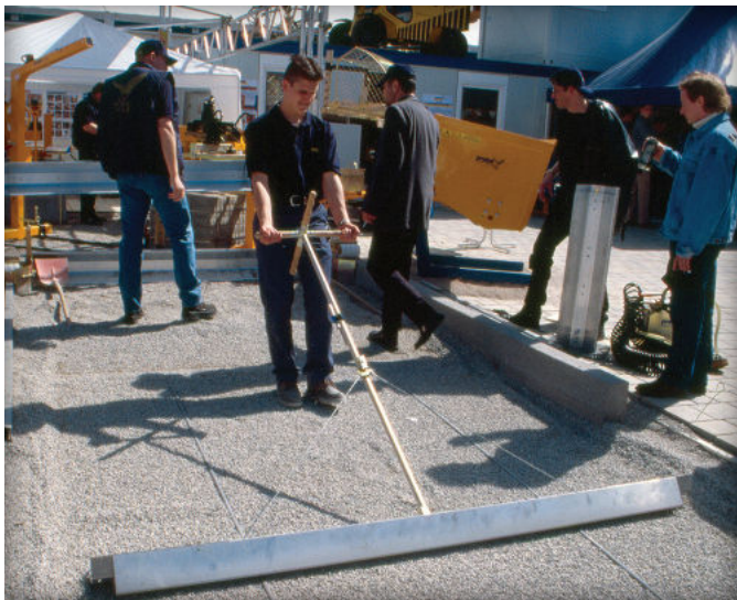
Figure 24. Manually screeding the No. 8 stone setting bed.
