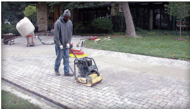
Figure 19. Edge restraint is spiked into the dense-graded base berms so it can hold the pavers in place during compaction and service.
