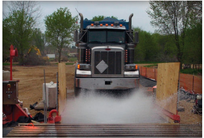
Figure 11. Larger PICP projects may require tire washing equipment for trucks to keep mud from contaminating PICP aggregates.
