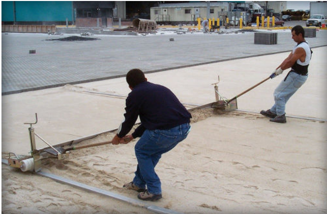
Figure 4. A two-man hand pulled screed
