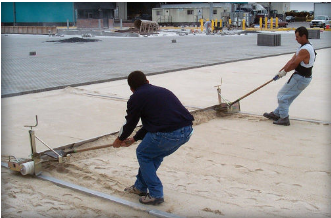
Figure 4. A two-man hand pulled screed
