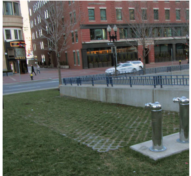
Figure 13. Concrete grid pavement typically reduces runoff in a manner similar to grassed surfaces and are best used to earn heat island reduction points.
