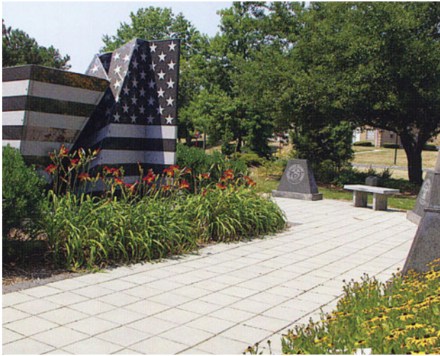
Figure 14. High SR paving slabs
