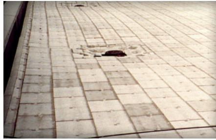
Figure 4. Some ballast-type slabs for roof decks are made with lightweight concrete materials. They can be joined with tongue-and-grooves and/or with connectors to resist wind uplift. This is one of several designs available.
