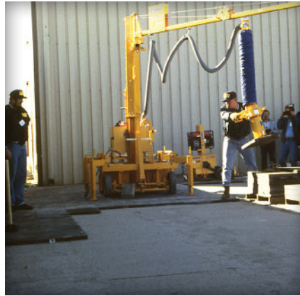
Figure 21. Vacuum assisted mechanical equipment for installing paving slabs.
