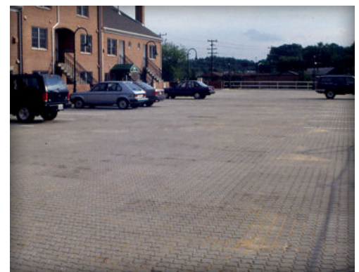
Figure 2. Concrete pavers serve vehicular traffic and parking over a concrete parking structure next to a residential development.
