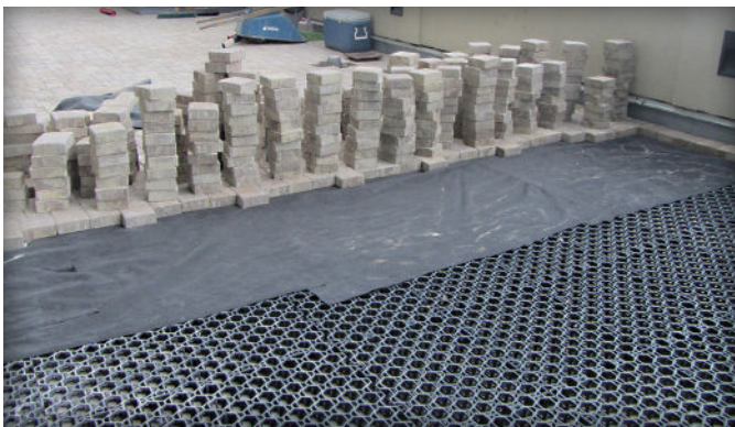
Figure 7. Concrete pavers on geotextile over plastic grids
