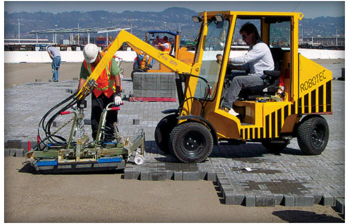
Figure 4. Hydraulic clamp picking up layer of pavers
