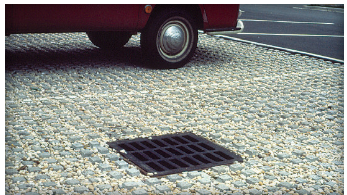
Figure 16. Concrete grids with aggregate in the openings
