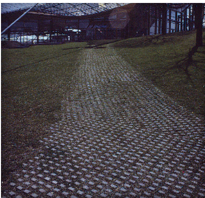
Figure 6. Service access lane
