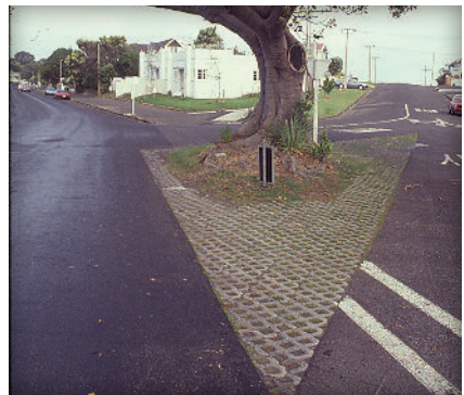
Figure 12. Air for tree roots and a warning for drivers
