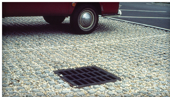
Figure 16. Concrete grids with aggregate in the openings
