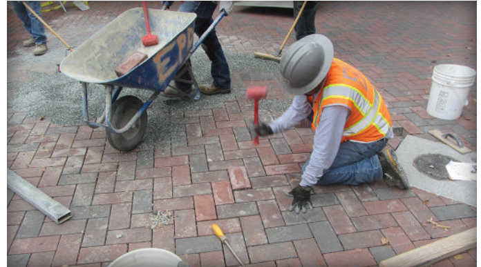
Figure 5. The final paver is inserted, the reinstated area compacted, joints filled, and compacted again. There are not cuts or damage to the pavement surface.
